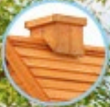
Wood Roof & Chimney
